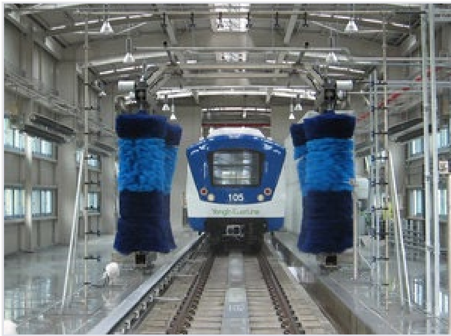
Diagram 6.9: Typical Automatic Train Washing Plant
